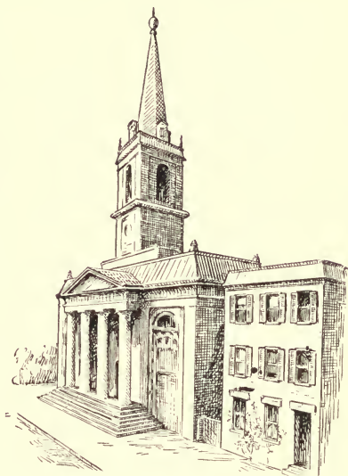
THE OLD CATHOLIC CATHEDRAL IN ST. LOUIS
